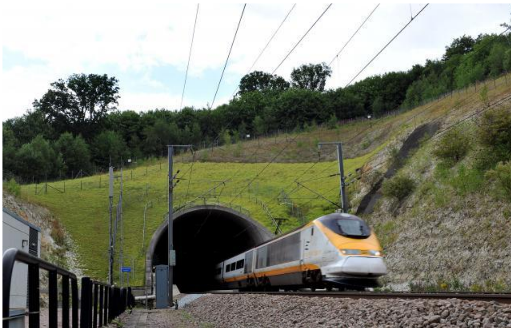
North Downs Portal
